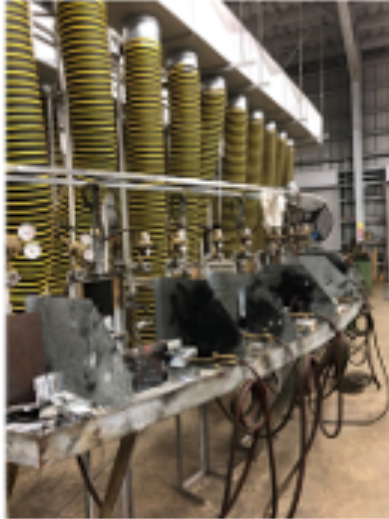
Welding Shop Oxygen and ACC Vent Area 2 Right Side
