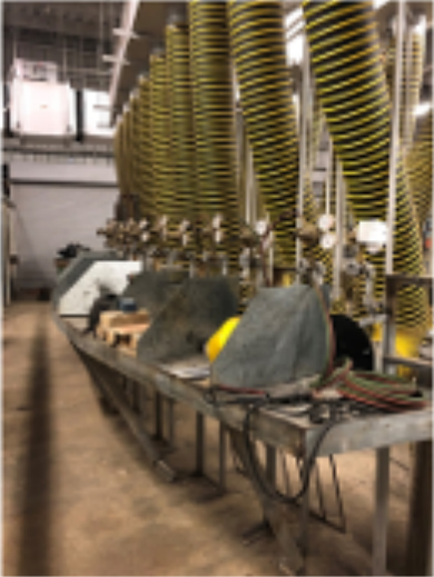
Welding Shop - Oxygen and ACC Vent Area 1 Left Side
