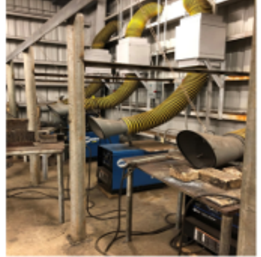
Welding Shop Oxygen and ACC Vent Area 3 Right Back Side (ARC)
