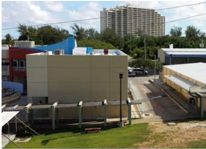
Overhead conduit at existing covered walkways will be converted to underground lines with the construction of new buildings and open space improvements.
