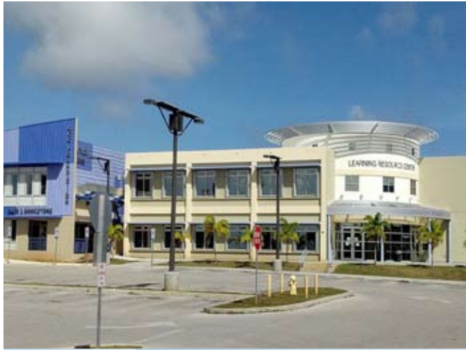
The Bookstore, Cafe, and Learning Resource Center create a "Student Services" core together with the Student Center at the Northwest corner of the campus.
